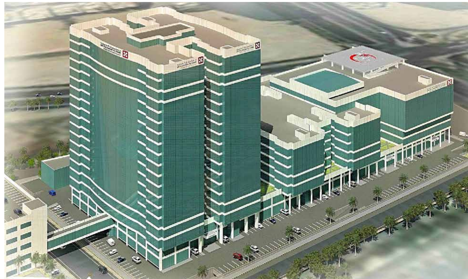
Dr. Sulaiman Hospital - KSA
